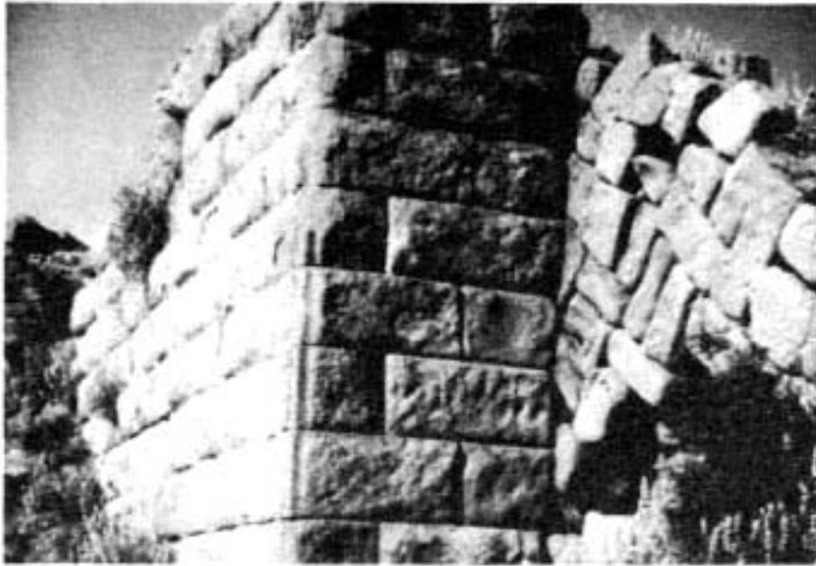
(a) Assos, Culvert in Fortification
